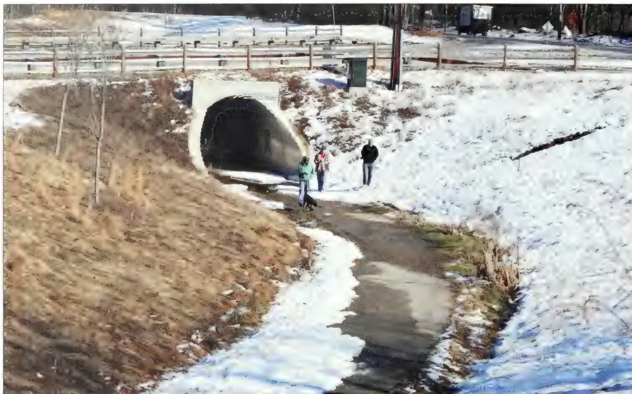
Figure 5.126. Example of a cut and cover tunnel routing the park "Battle Road Trail" below Hanscom Drive, Minute Man National Historical Park. This type of tunnel, installed from prefabricated segments, is under consideration to provide visitor access to one of Sandy Hook's subsurface NIKE missile magazine rooms (January 2009, Minute Man NHP, Massachusetts).
